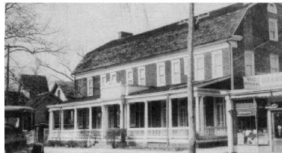
The exterior of Matinecock Lodge in February of 1933. To the left is Raynham Hall prior to its restoration.>
