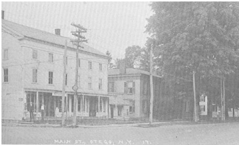
Business block at the corner of River and Main streets is occupied by the Warren Wilbur general store, and the Masonic and Eastern Star lodge rooms on the second and third floors..
